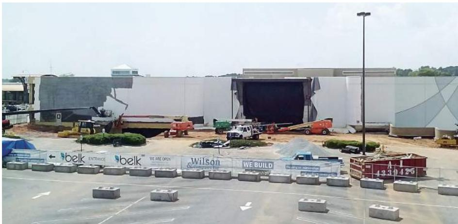
*Belk Store in Greenville, S.C., where Wilson & Company is under contract with repeat client Belk Stores to demolish and rebuild the exterior of the building. This project involves deep excavation, new entrances, and new exterior finishes, all being accomplished while the store is open for business.*
